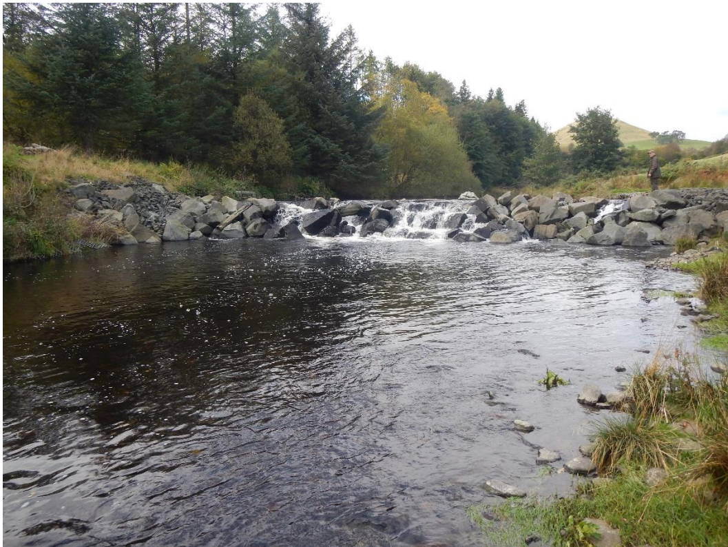
Figure 17. The weir that feeds the fish farm is likely to be impassable by fish in most flows.
