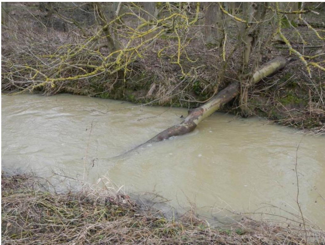
Figure 21. A lodged flow deflector – the technique can be used with a single trunk or branch (primarily to increase scour) or a multi-branched limb (to create greater flow dissipation and more in-channel structure). The elevated butt end (bank end) reduces the potential for detrimental bank scour (usually associated with d/s deflectors) as a through-flow is maintained along the bank.
