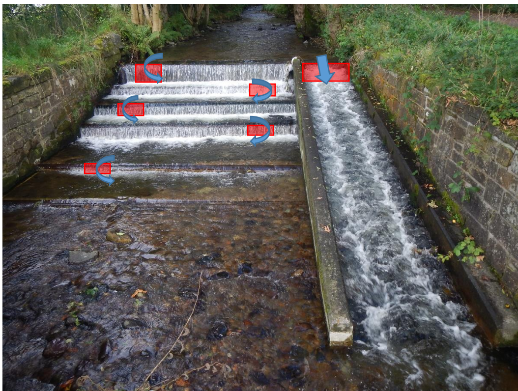
Figure 23. Possible notching of the weir that could reduce the potential for super-charging the Larinier pass with flow by the required crest lowering at the upstream end. This option would actually improve the passability of the weir via an alternative route, delivering multiple benefits. The blue arrows signify the potential flow pathway though the notches.
