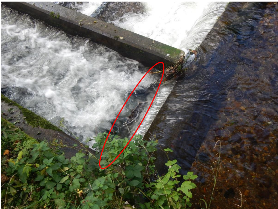
Figure 20. The significant step and thin film of water, with air cavity behind, falling onto the top baffle of the Larinier pass (red ellipse) creates a major obstruction to further upstream progress for fish.
