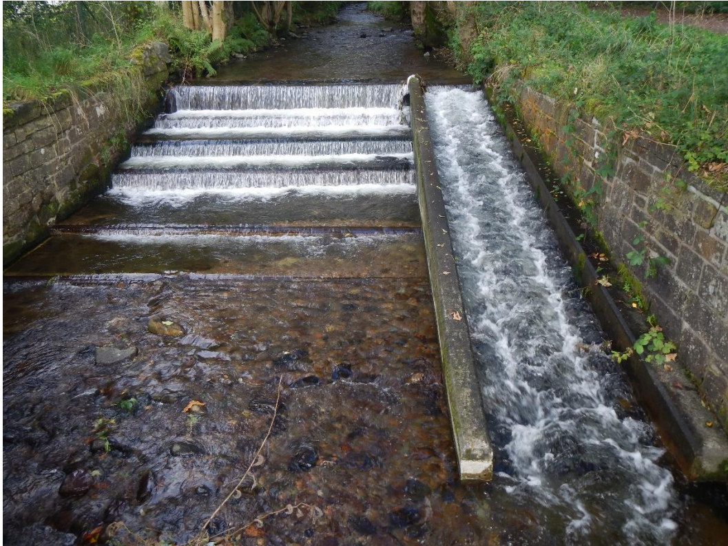
Figure 19. Looking upstream at the weir, with stepped pools and a poorly installed fish pass to the LB side (right of shot).
