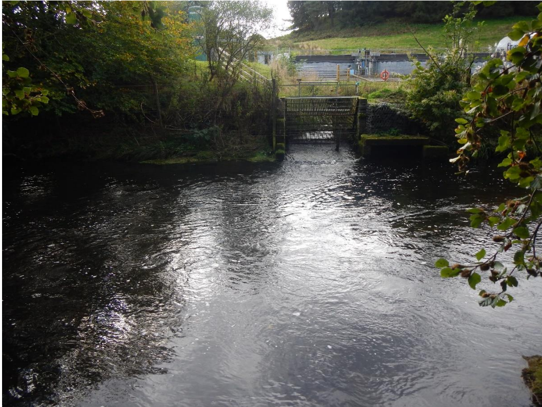
Figure 15. The outlet to the salmon rearing unit. The coarse screen should prevent the escape of larger fish, but much finer screening should also be in place within the farm to retain juveniles.
